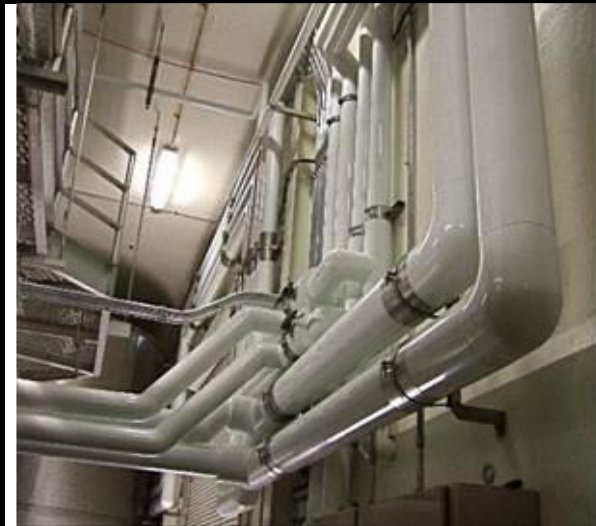
Hot Pipe Insulation with GRP Cladding
